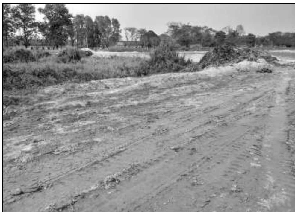
Earth-filling activities under way at GU Campus
